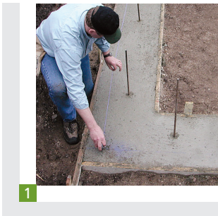
1 Prepare the job site
